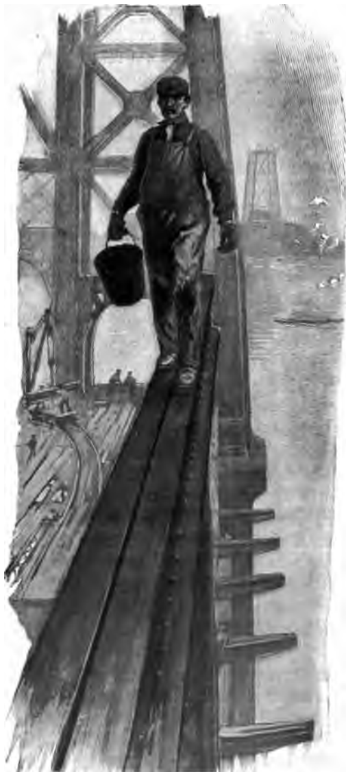
WALKING A GIRDER TWO HUNDRED FEET IN AIR.
